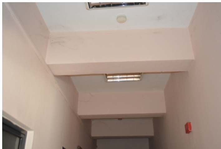
Photo 6 _The hanging beams of the building
